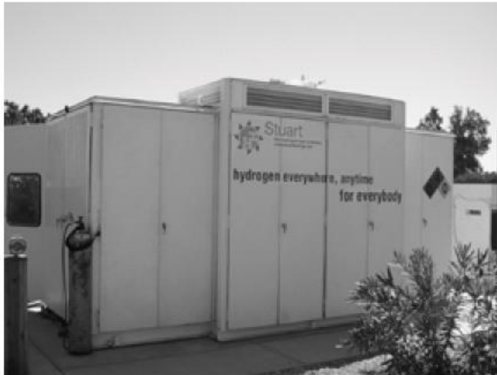
Stuart Energy's modular compressed hydrogen station
